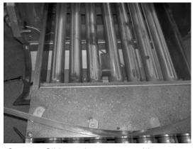
Step 14: Slide out burner assembly
